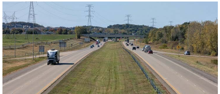
Photo credit: Matt Zeller, Concrete Paving Association of Minnesota
